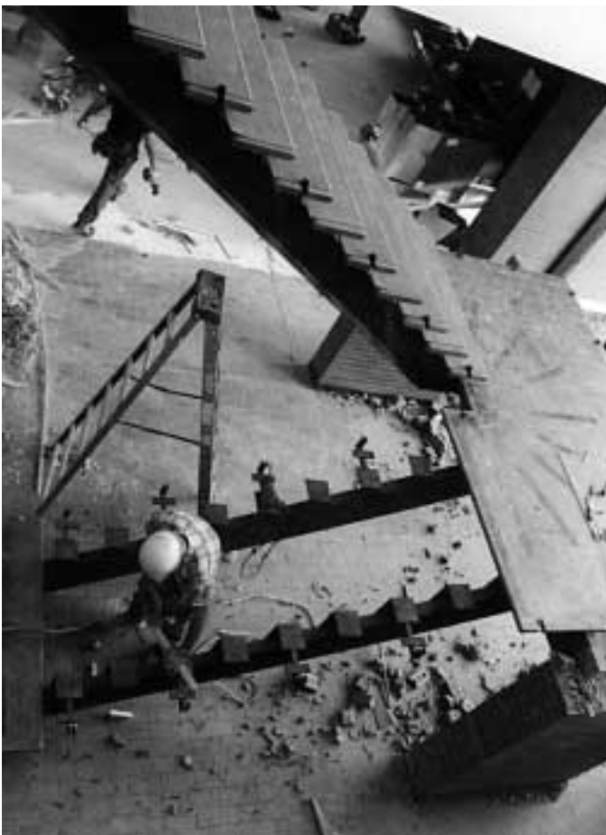
The central staircase to Resnick Library was removed as part of the recent renovation. The vacated space allowed for the installation of a café and an ideal view of the valley.
